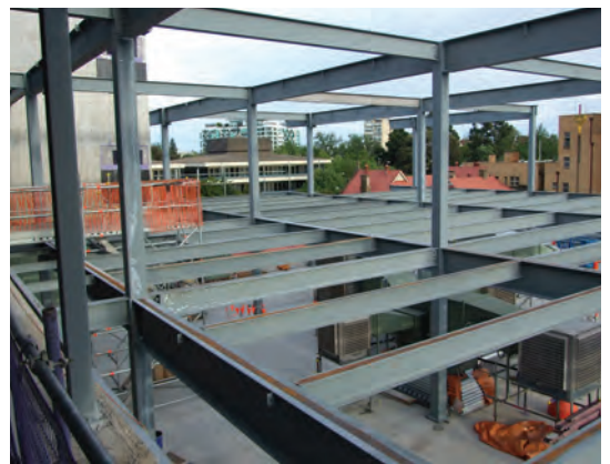
The structural steel framework to level 7.
