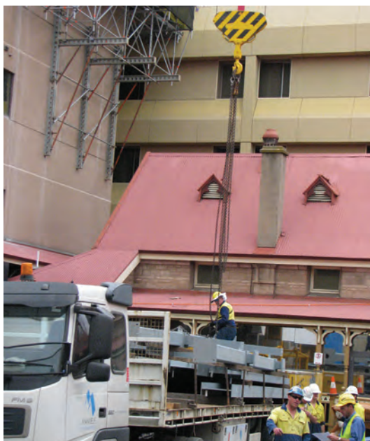
Preparing to lift some materials with the crane.
